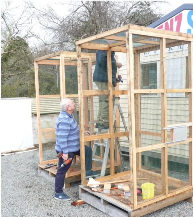
Trial assembly of the flat-pack aviaries that the shed builds for the DOC Orange-fronted parakeet program. The aviary packs are lifted into the bush by helicopter.
